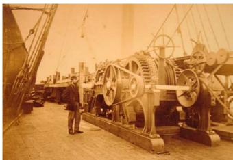
avoid twisting or stressing it, otherwise it could snap or split, go open circuit or allow salt water in. Obviously crossing the Atlantic involves laying down huge amounts of cable vertically from the ship to the sea floor. These had to be supported by giant buoys, gradually removed as progress was made, without them (and sometimes with them), the ship was very unstable. Since the goal was to lay these single stretches there was no opportunity to return to port, it was a
